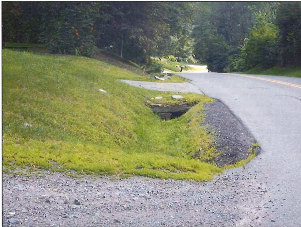
Photo 5. Photo shows stone drainage feature and gully on the upper portion of Church Street. View is to the north.
