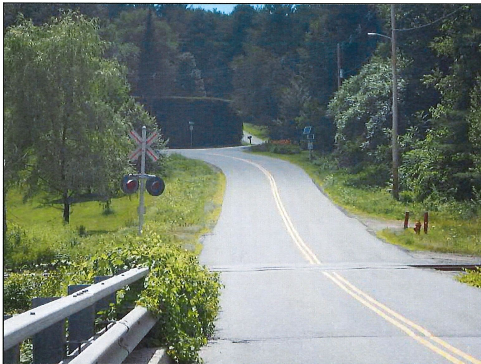
Photo 7. Photo shows the slope leading down to the railroad and Williams River valley. The railing of the bridge over the Williams River is visible in the foreground. View is to the southwest.
