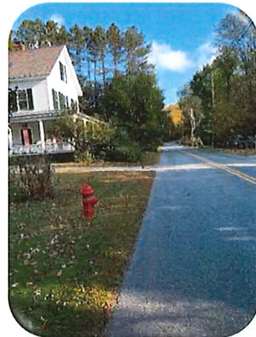
Existing Hydrant along Church Street
