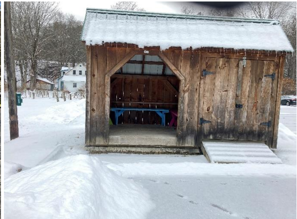
Shed to be moved
