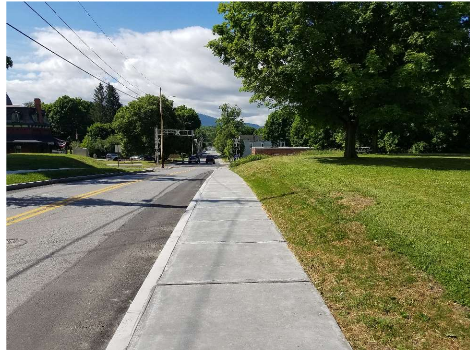
Sidewalk w/ Curb
